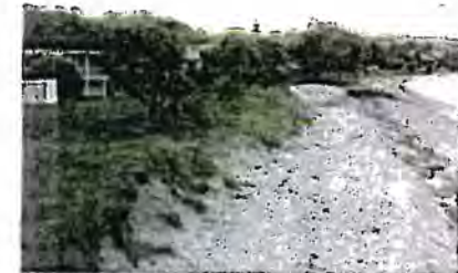
Coastal erosion will continue to be an issue along the foreshore during periods of high seas. The esplanade Reserves in this area have almost disappeared.
