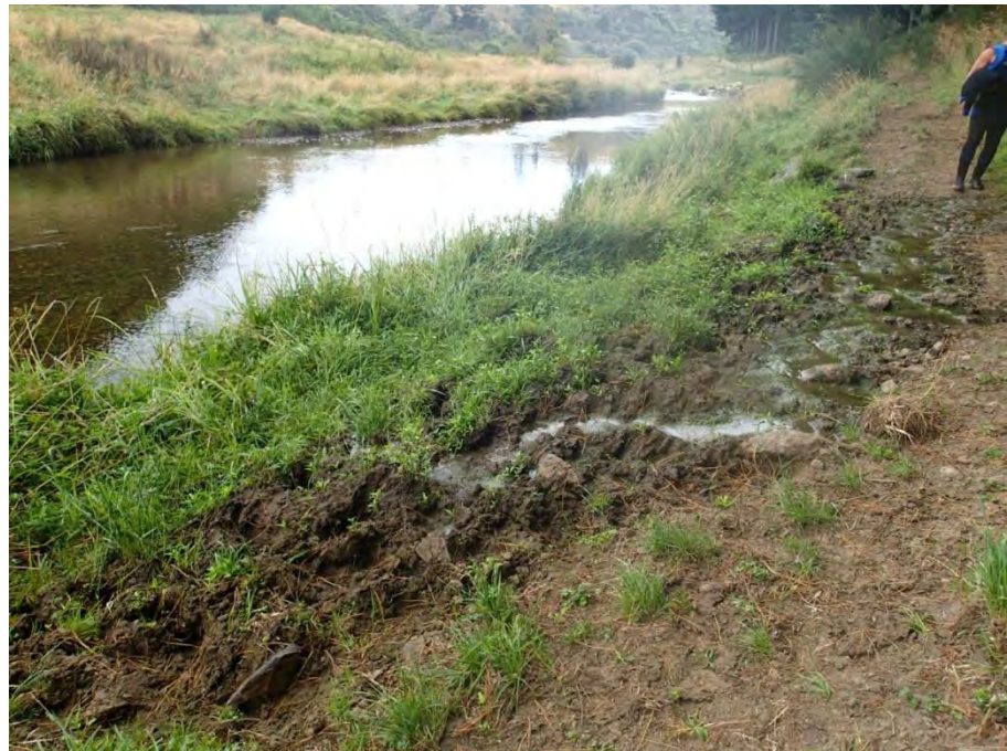
4.5.11 Figure 2. Unfenced marginal strip converted to a dairy race with no sediment trap on Mangatutu Stream bank, first used in approximately 2013.
