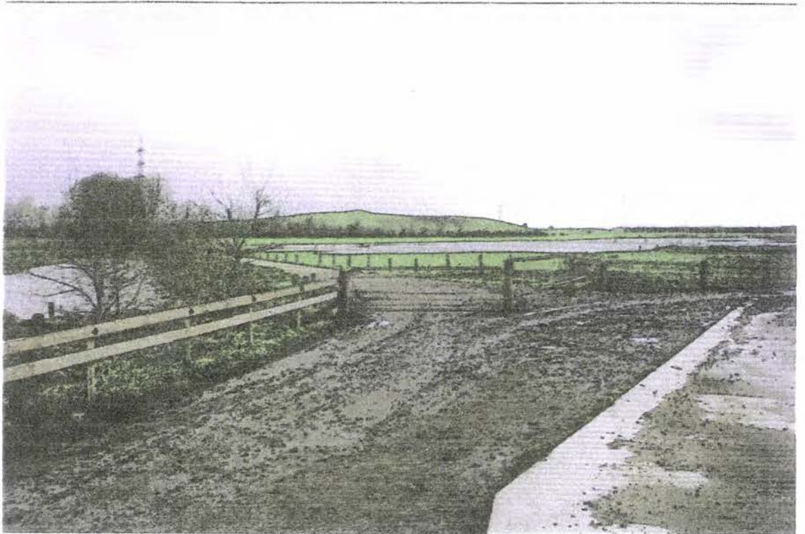
WUA built step bank with drain elements.
