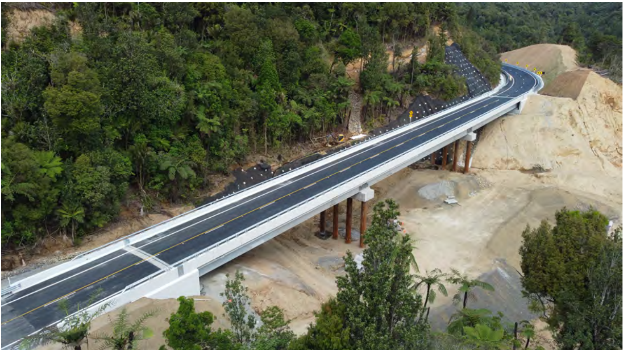
State Highway 25A Taparahi Bridge. Image courtesy of NZTA
