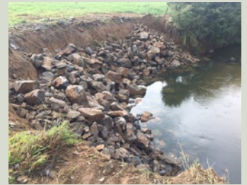
Rocks used to stop erosion. Summer 2017/2018.
