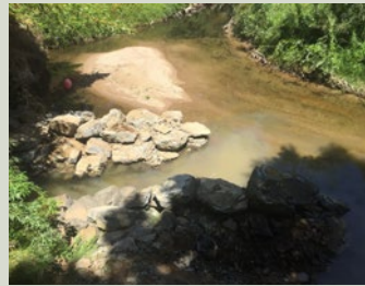
Groynes installed for erosion protection along the river bank. Summer 2016/2017.
