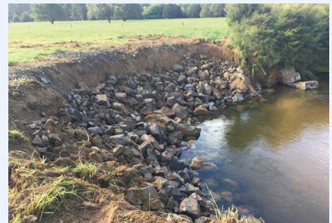
The rock armouring in place, with followup planting to occur.
