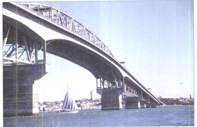
Auckland Harbour Bridge.
