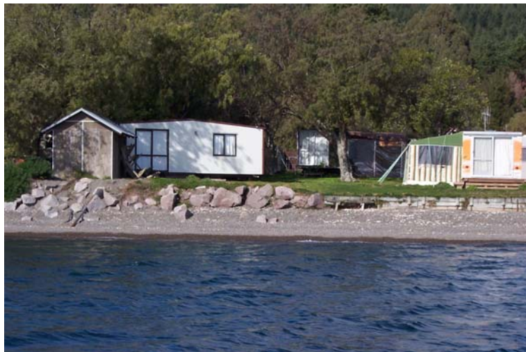
Photo 9. Motutere rock wall and wooden structure mix, August 2005
