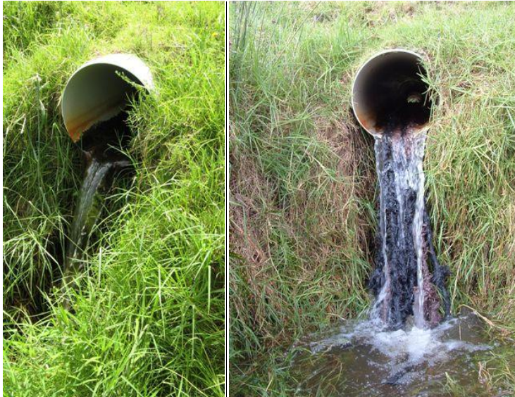
Lake Harihari culvert before (left photo) and after (right photo). Installed for improved eel passage in 2009 following a netting survey which suggested poor recruitment of elvers to this lake. Assessment of the effectiveness of this retrofit is planned to occur in 2015.
