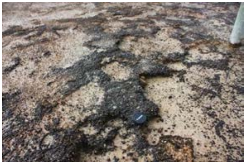
Plates 77 and 78: Deteriorating sinter terrace. Structure still visible but very brittle/soft underfoot at Feature 1, Wharepapa Road.
