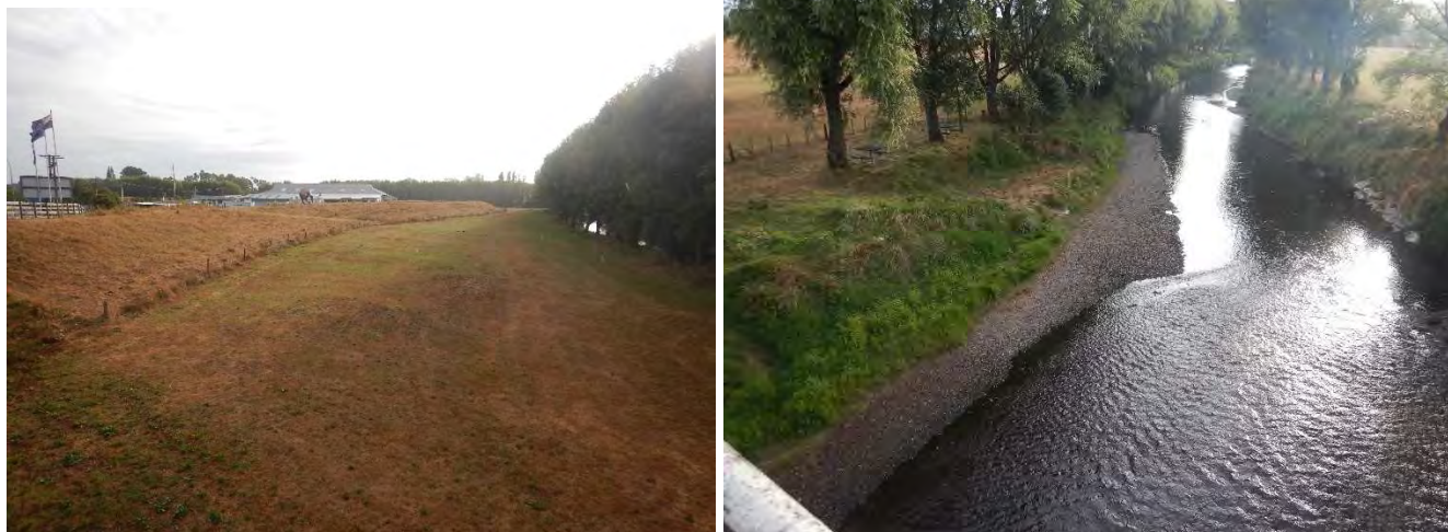
Figure B.44. Photographs showing features (stopbanks, left) and a representative reach (right) of the PC_SBkMC_DcFp_Gbed River Style along the Waipā River at Ōtorohanga.
